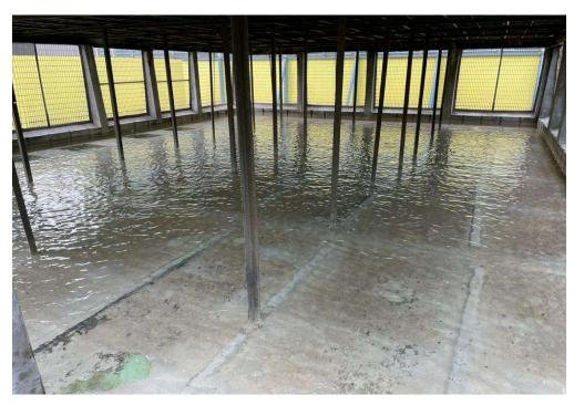
Take Away:- 8 weeks post commissioning of the SBR cooling towers became completely clean with no signs of Scaling, Fouling & Corrossion
